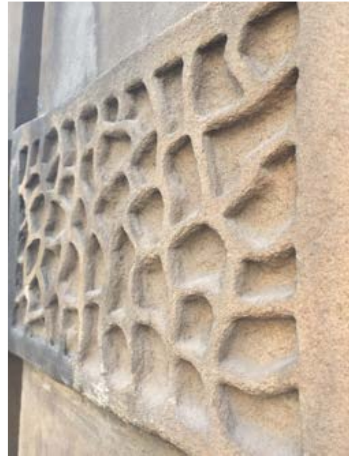
Wall at the back of the Wellgate Shopping Centre.
